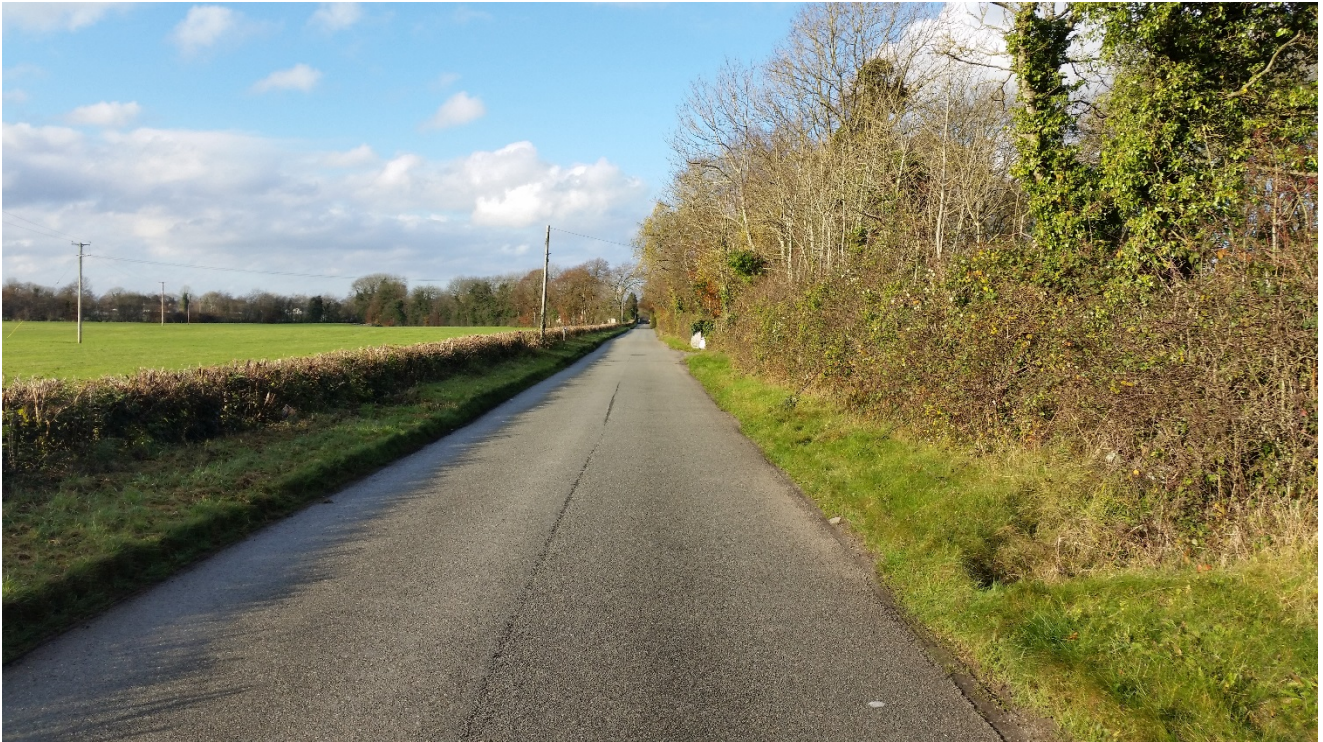
Figure 3.11: View northwest of proposed location of access road to T47
