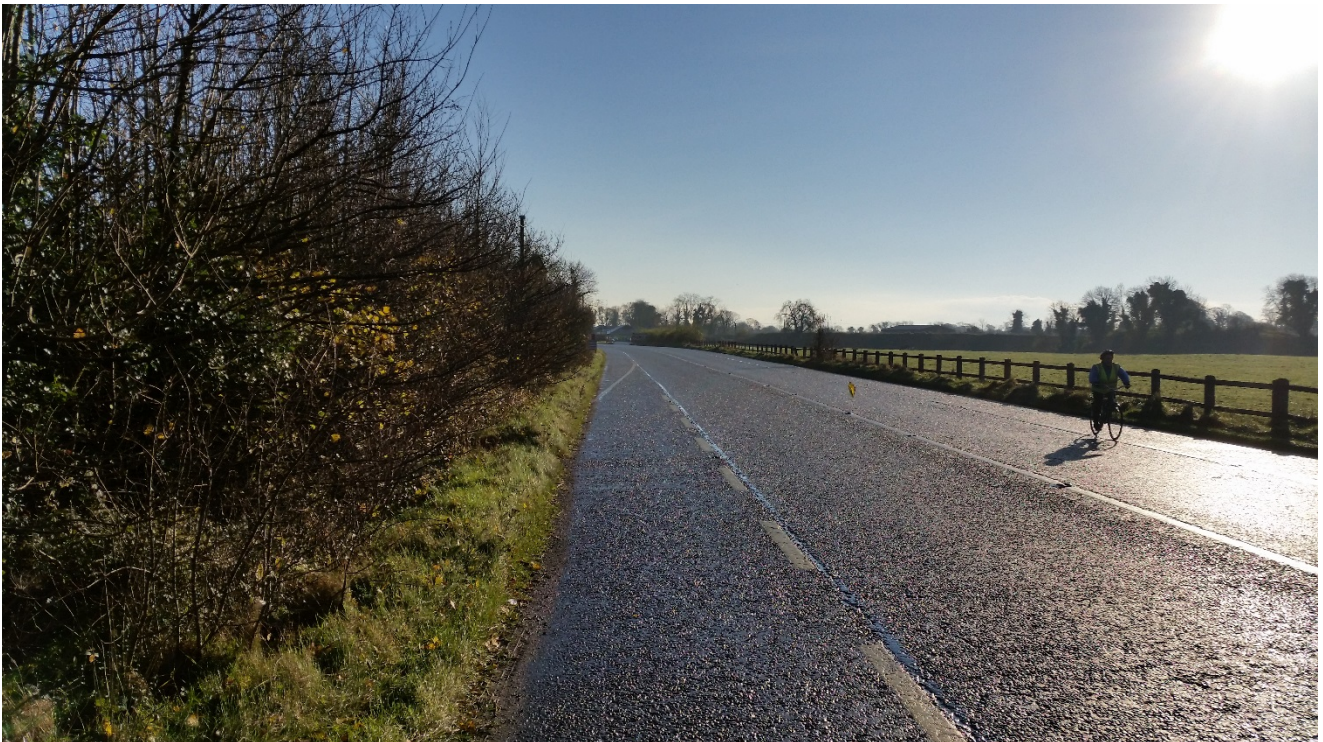
Figure 3.3: View east from the existing southwest access to Ballynakill Cluster
