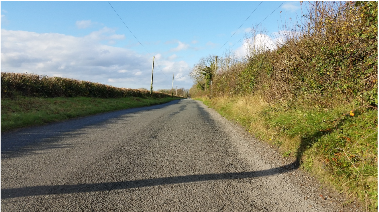
Figure 3.15: View northwest of proposed location of access road to T11 to T23
