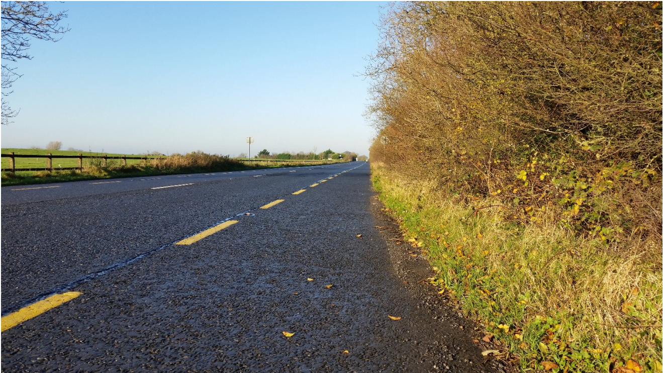
Figure 3.2: View west from the existing southwest access to Ballynakill Cluster
